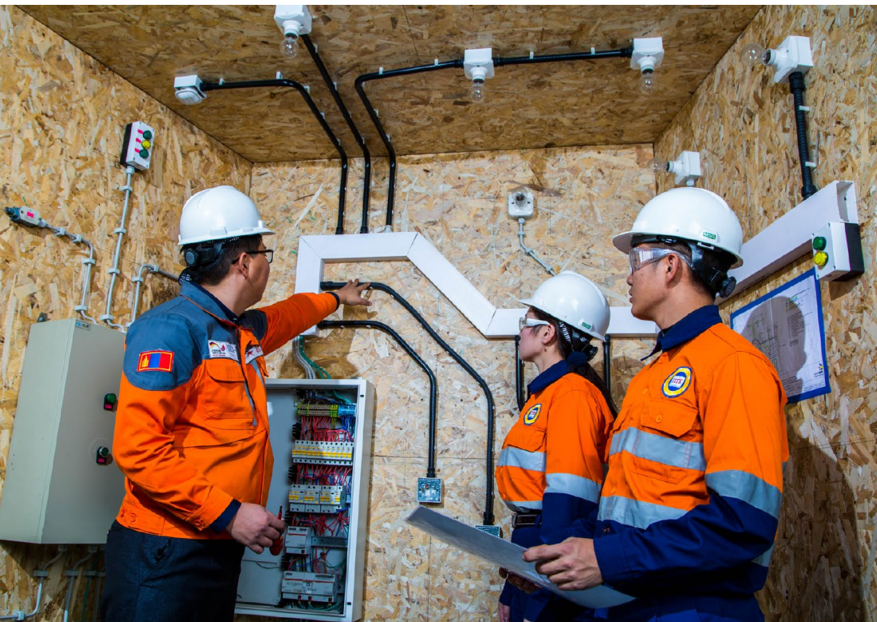
Electrical training at a TVET school in Darkhan-Uul, Mongolia. © GIZ Mongolia
