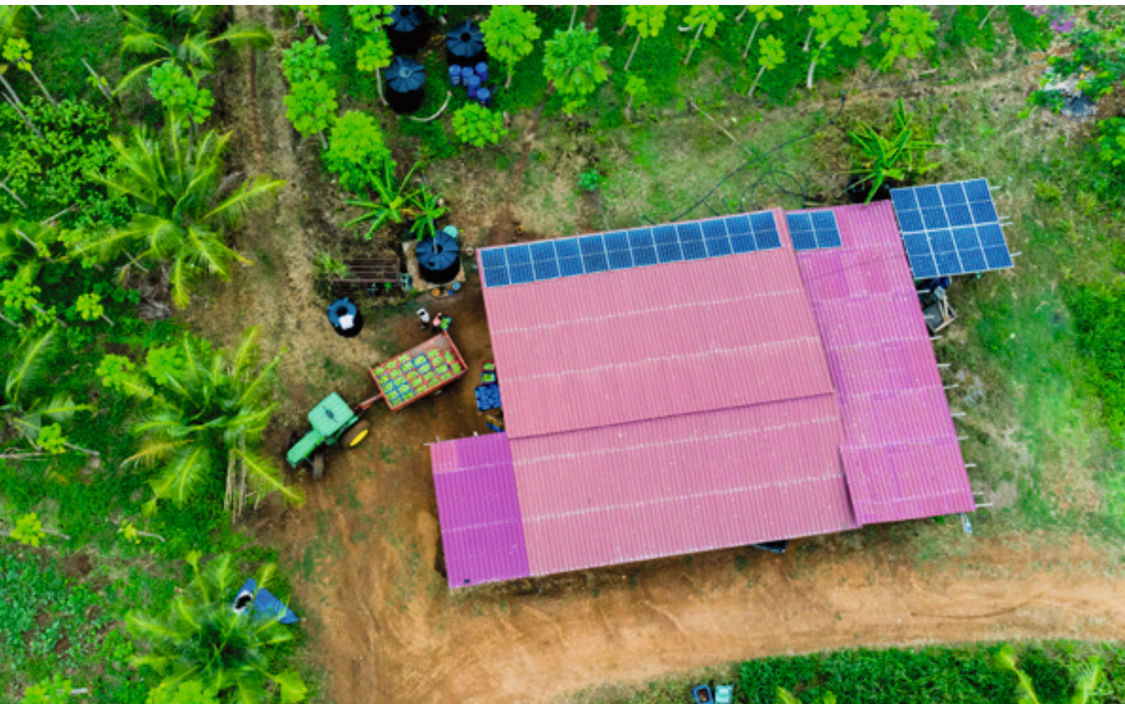
A farm in Ghana using solar energy for irrigation – supported by GIZ's Green People's Energy Project. © GIZ
