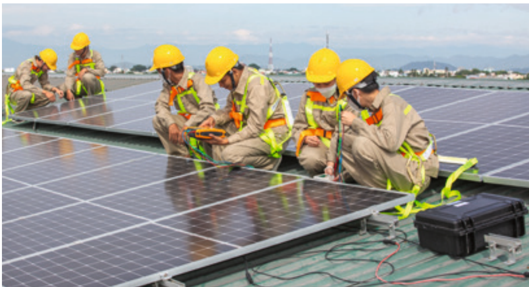
Ninh Thuan Vocational College trainees perform measurements on PV panels during a practical training session. © GIZ Vietnam/Nguyen Ngoc Quang
